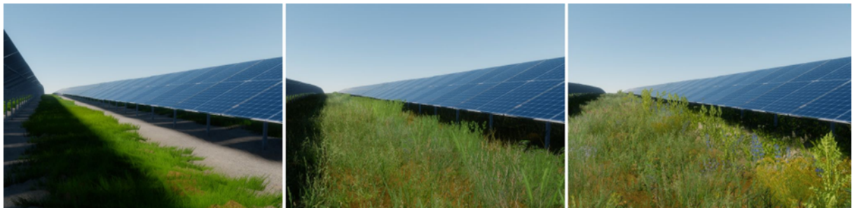
Figure 6: Visualization of different management methods of PV fields: intensive (left, graveled and regularly mowed, distance of 2m between modules), medium (center, mowed and mulched, 4m between modules), and extensive (right, measures taken to promote flowering plants, 6m between modules).
